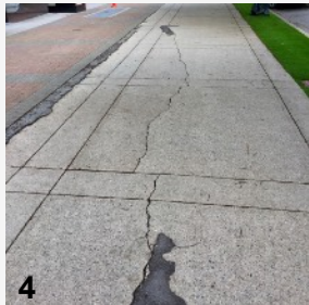
Concrete that has cracked
